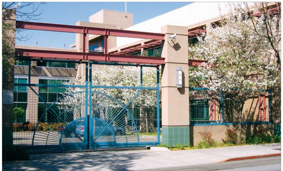
A decorative gate and fence screen a parking lot in Berkeley, California.
