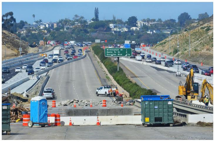
Interstate 5 traffic in Encinitas is diverted in the spring of 2020 as crews work to demolish the old bridge over San Elijo Lagoon.
