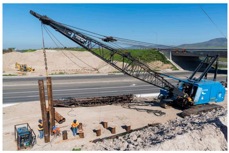
Caltrans and SANDAG crews install piles just south of Otay Mesa Road to support the new SR 11 connector ramp to SR 125.
