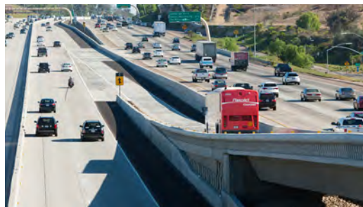
Direct Access Ramp (DAR) A special highway entrance where buses, carpools, or people who pay a toll can directly enter managed lanes without having to merge from the right side.
