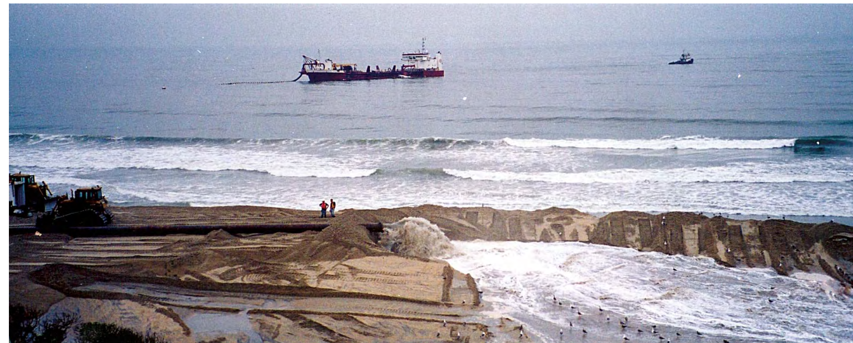
Photograph B: Slurry Discharge and Training Dike
