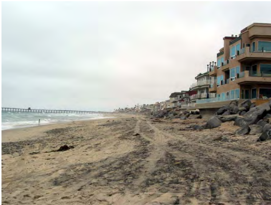
Photograph A: View looking north near Descanso Avenue
