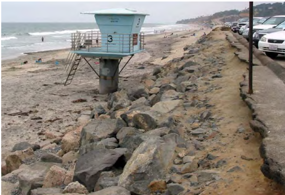
Photograph B: Rip-rap protection along North Torrey Pines Road
