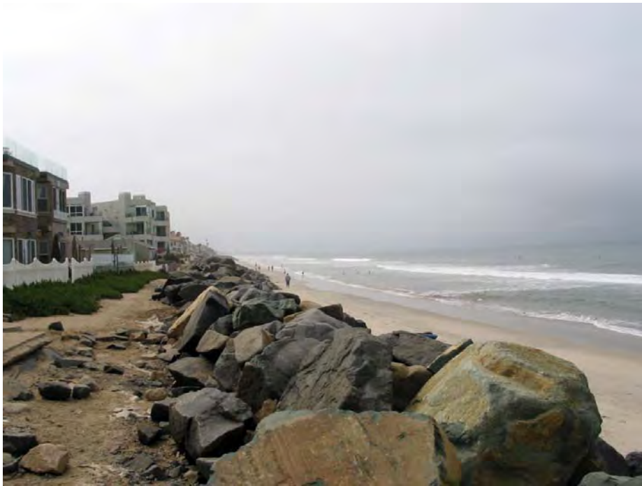
Photograph A: Typical rip-rap protection
