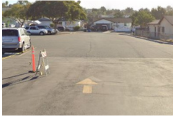
Figure 3. Traffic direction arrows are missing on one half of the school parking lot.
