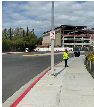
Figure 5. Bike lane is not painted.
