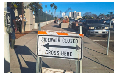
Figure 3. Sidewalk closed and tents on bridge overpass at the corner of Orange Ave. & 40th St.
