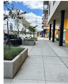
Figure 1. Upkept sidewalk in front of affordable housing complex along Imperial Ave. between 63rd St. and 64th St.
