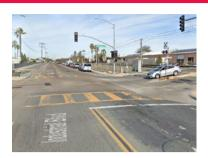
Figure 6. Faded crosswalks on the corner of Industrial Blvd. & Naples St.
