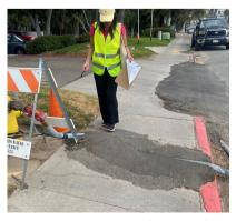
Figure 6. Pipe coming from the fire hydrant that has been paved over disrupting the sidewalk and curb
