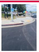
Figure 3. Needs additional curb cut (SW and SE corners of Euclid Ave./Market St.)
