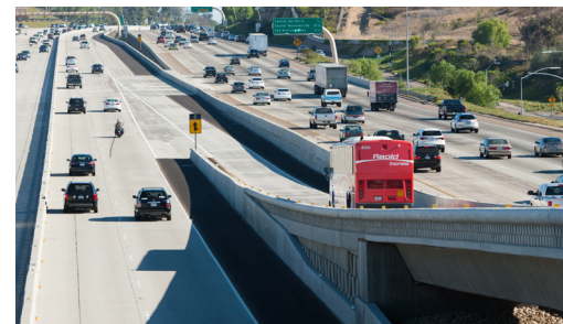
Direct Access Ramp (DAR) A special highway entrance where buses, carpoolers, or people who pay a toll can directly enter managed lanes without having to merge from the right side.
