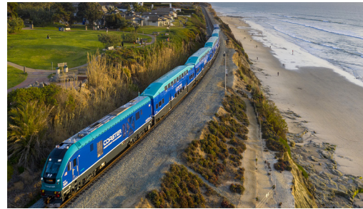
LOSSAN Improvements Making the railway that connects San Diego to Los Angeles and San Luis Obispo safer, faster and more efficient.
