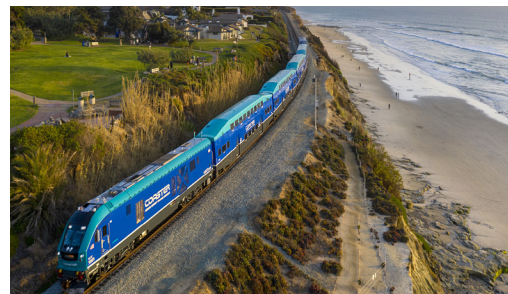
LOSSAN Improvements Making the railway that connects San Diego to Los Angeles and San Luis Obispo safer, faster and more efficient.
