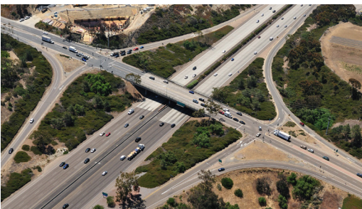
Highway Intersection Improvements Improves safety, and traffic flow in places where a highway crosses a major road.
