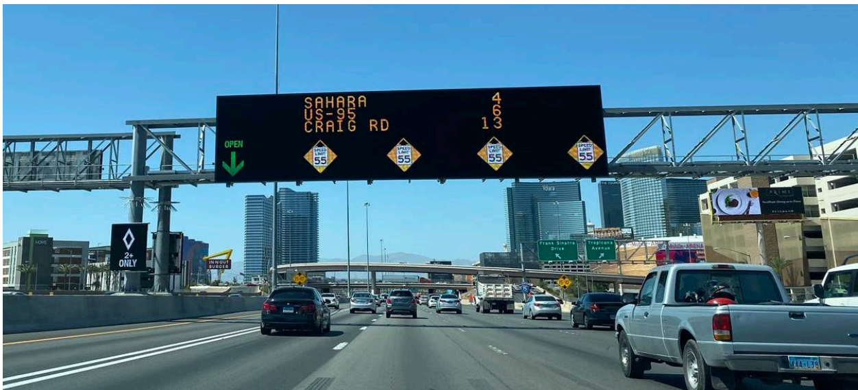
Active Traffic Management through dynamic speed limit and lane assignment signage along I-15 through Las Vegas.
