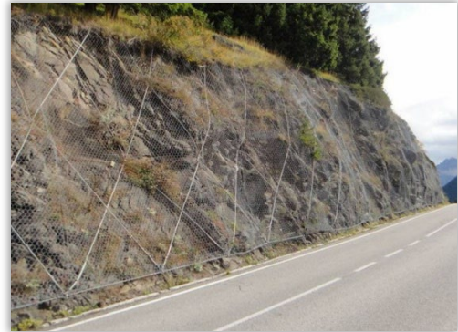
Photo Source: Shandong Xingying Environmental Energy Technology
