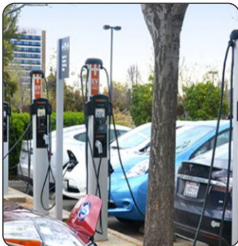
Electric Vehicle Charging Stations
