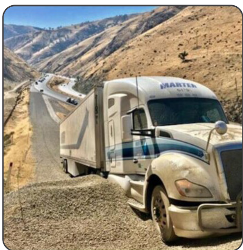
Runaway Truck Ramp
