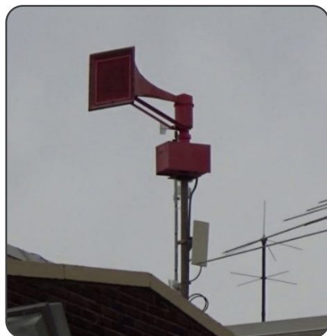
Emergency Evacuation Siren
