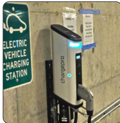
Electric Vehicle Charging Stations
