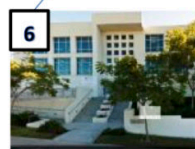
Villanueva 1901 Del Sur Blvd., 2nd Floor
